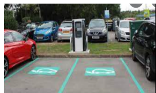
Communal EV charging points
